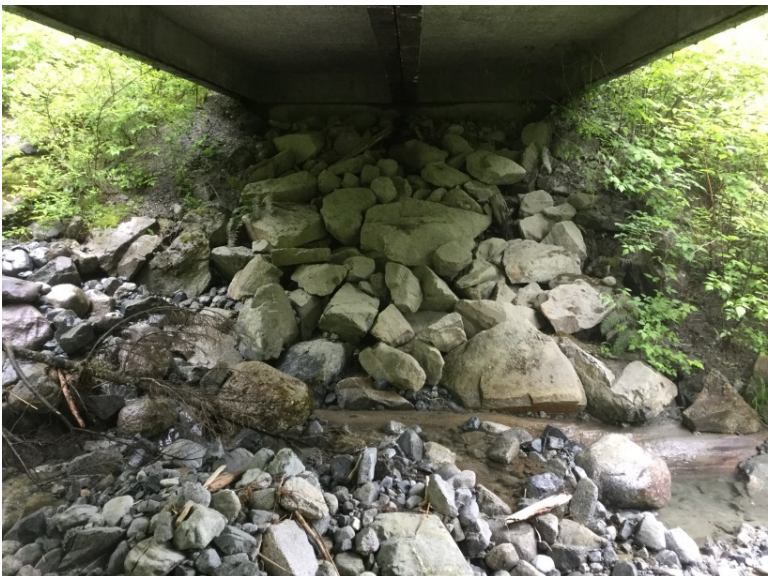
Left Bank Abutment when facing downstream
