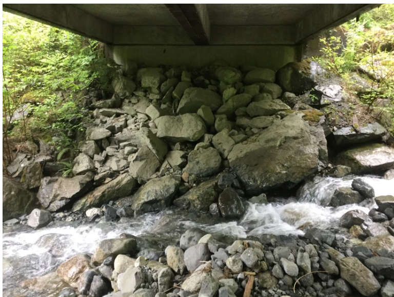
Right Bank Abutment when facing downstream
